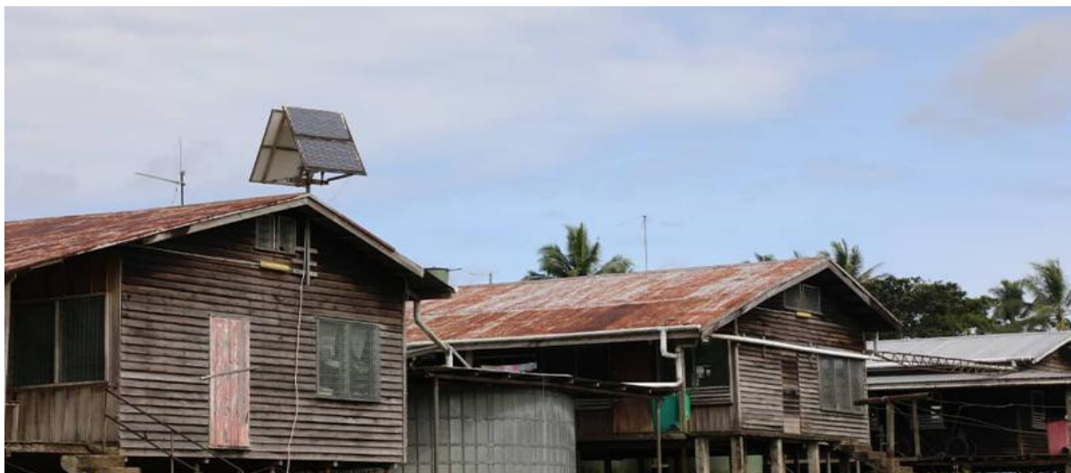
Inserted: Western Province, North Fly, ECPNG - Rumginae Rural District Hospital
