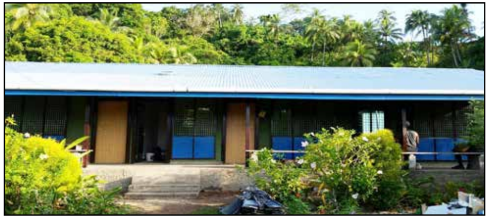
Maintenance of the Kabanut Health Centre is an achievement for the community
